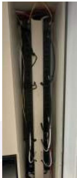
All electrical energy in the system is distributed via 2 **Canovate IP PDU 20xC13 4xC19 SOCKET 3xCIRCUIT BREAKER PDU LEVEL 32A 3mt COMMANDO PLUG**. These PDUs can be connected to the meeting table via the LAN line and controlled via software.
